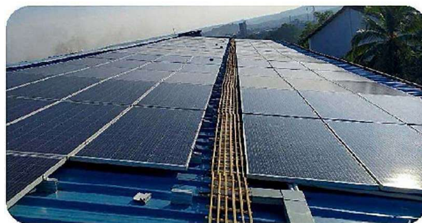
Solar Panels are installed at Roof top of Mysuru of capacity 164 kW
